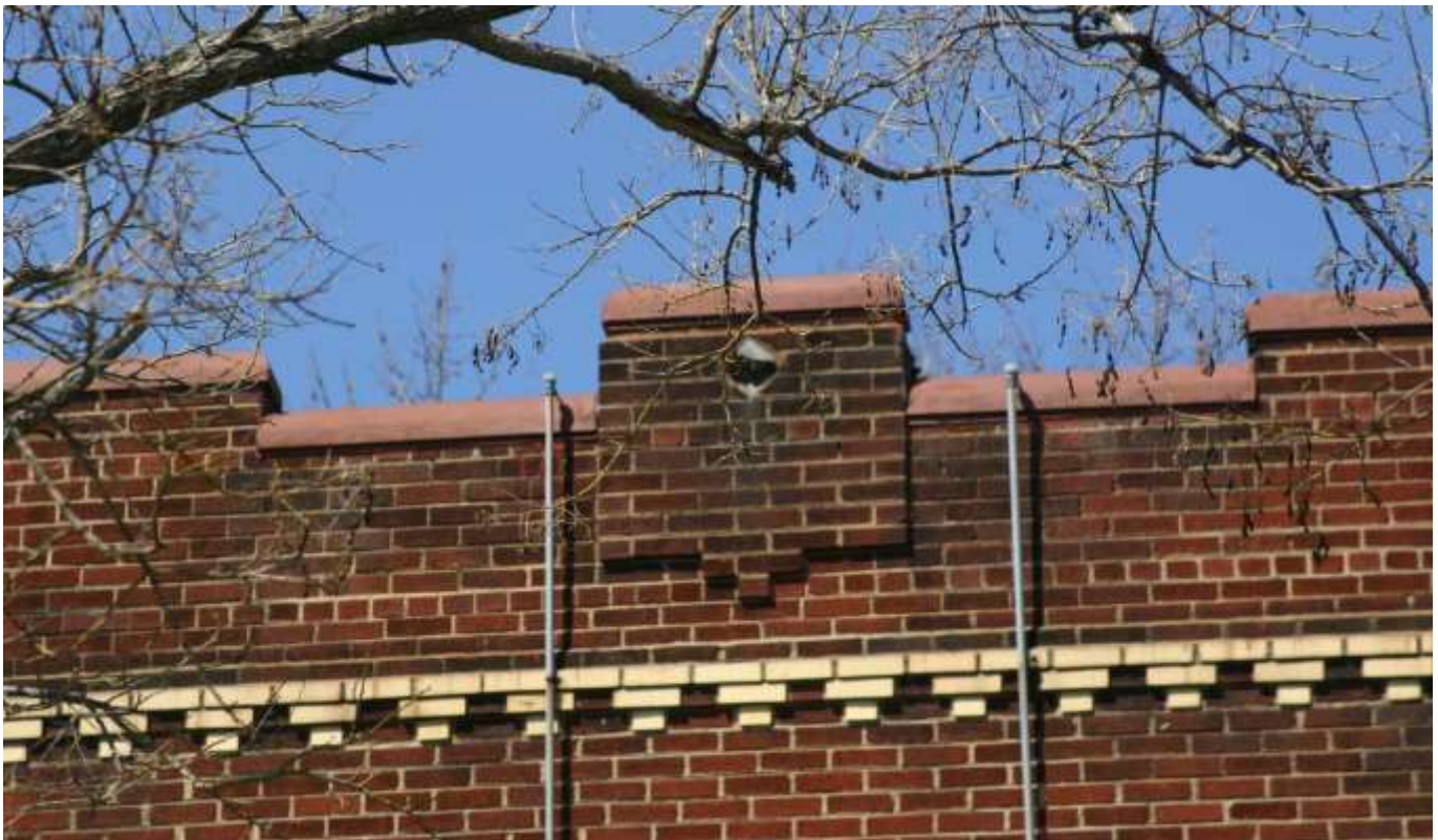
4. 422 E. Glendale Avenue. Facade (south elevation), detail: glass block in central parapet keystone, straight angle, facing 350° N. Photo by Gwen White 4/6/2014.
