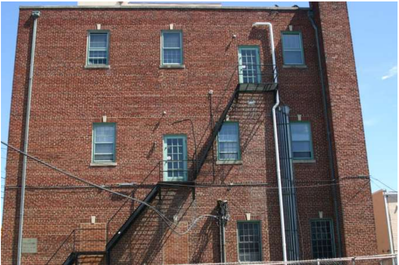
6. 1908 Mt. Vernon Avenue. Rear (west) elevation, straight angle, facing 78^{\circ} E. Photograph by Gwen White, 4/6/14.
