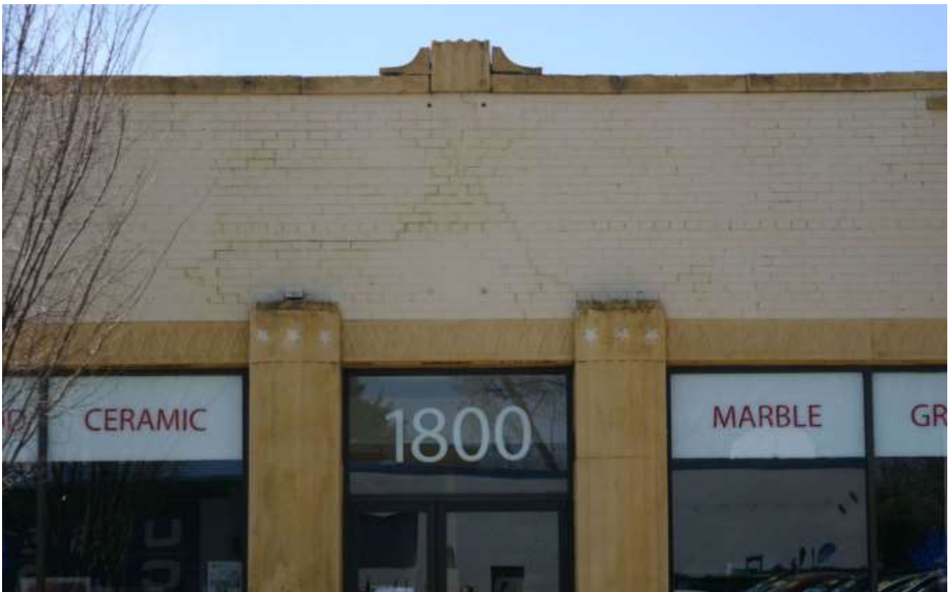
2. 1800 Mt. Vernon Avenue. Facade (east) elevation, detail entrance pilasters, straight angle, facing 268 0 W. Photograph by Gwen White, 4/6/14.
