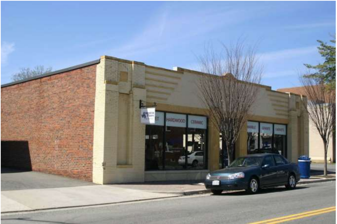
5. 1800 Mt. Vernon Avenue. Façade and front half of south elevation, oblique angle, facing 291 0 W. Photograph by Gwen White, 4/6/14.
