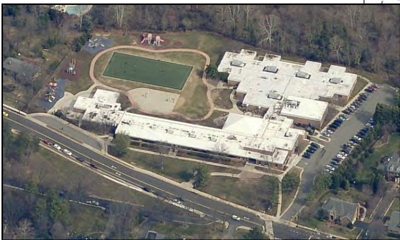
School site looking north across Janneys Lane
