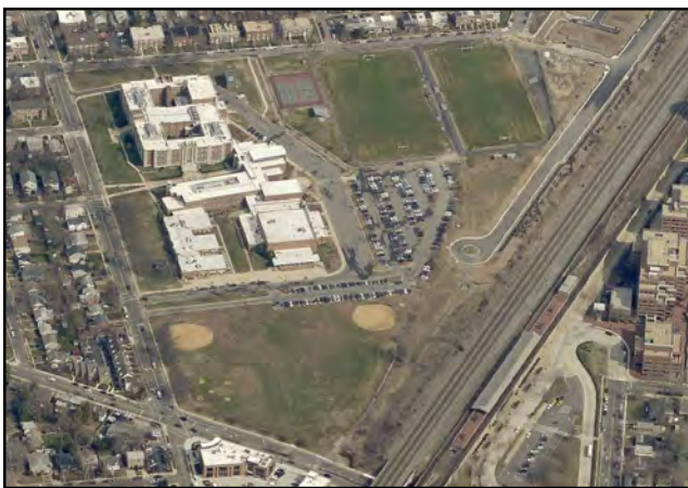
School site looking north across Braddock Road and the Metro and CSX rail lines. The Braddock Road Metro Station is at the lower right.
