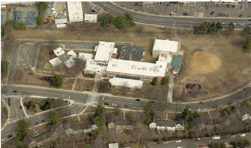
School site looking north across Martha Custis Drive.
