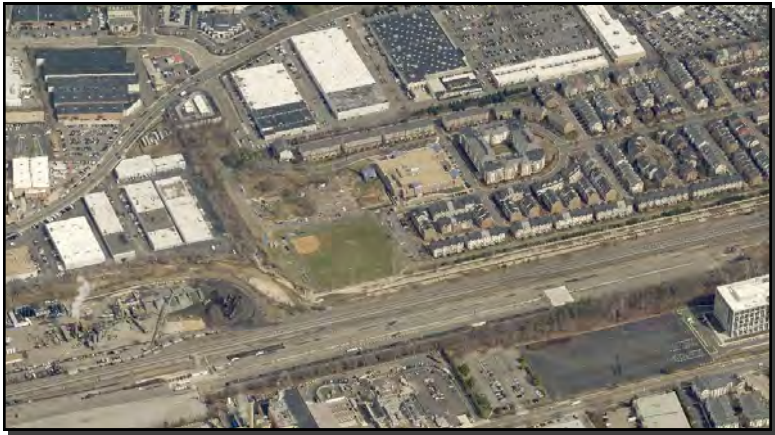
Neighborhood context. The Norfolk Southern tracks and Cameron Run separate the site from uses along Eisenhower Avenue, shown at bottom right in this photo. Pickett Street runs along the upper left. The Cameron Station residential development is to the right of the school.
