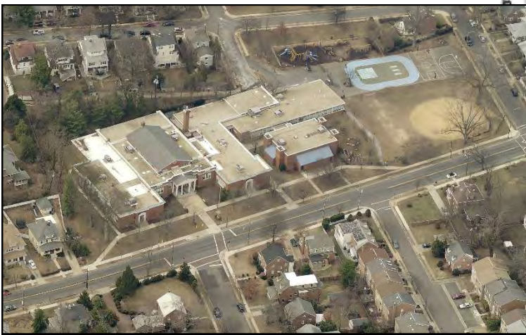
School site looking west across Russell Road
