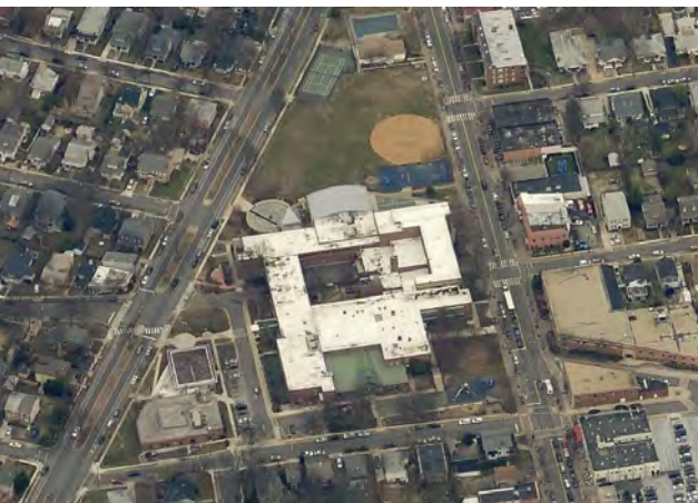
School site looking north. Commonwealth Avenue is on the left, and Mount Vernon Avenue on the right. Duncan Library is at the lower left.
