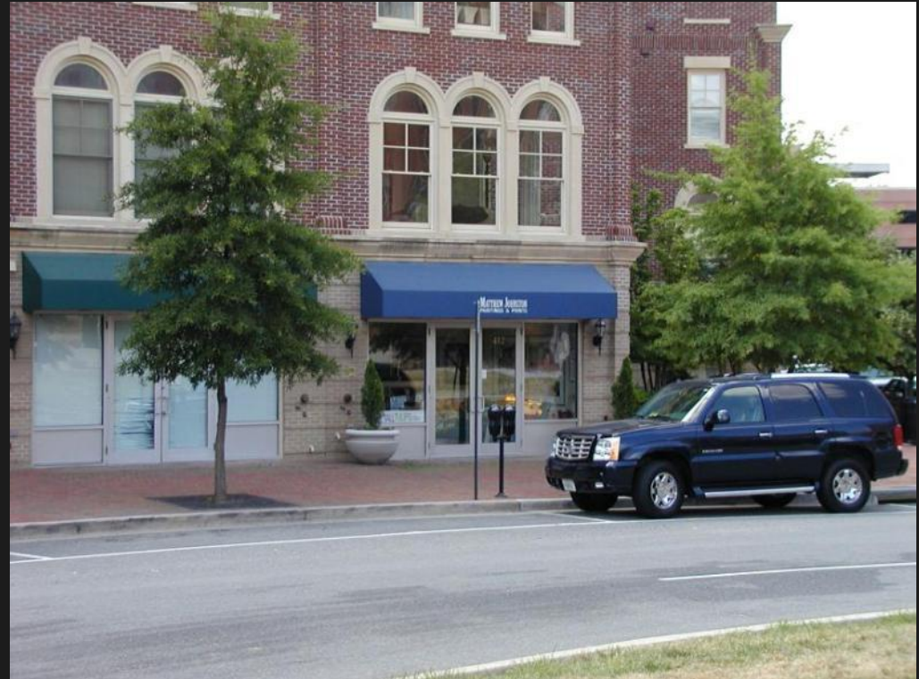
Block H Townhouses – John Carlyle Square Frontage
