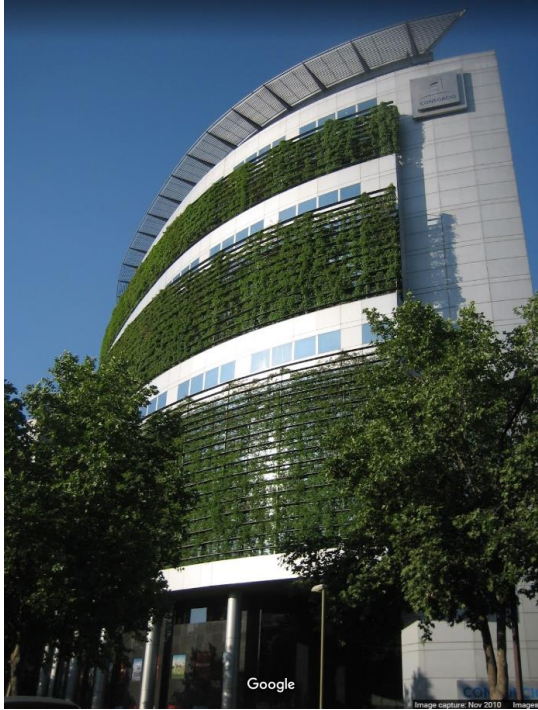
Edificio Consorcio | Santiago, Chile | Green Screening (Figure #5 above)
