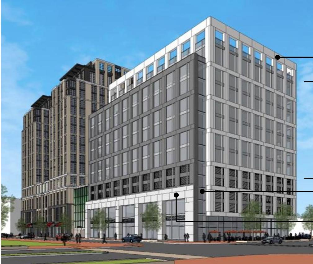
PREVIOUS 7 Floors of Medical Office Building
