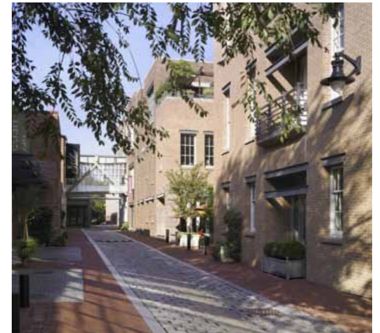
Pedestrian-friendly service court
