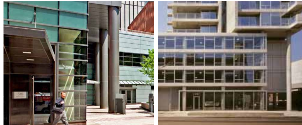
Building base with “Pilotis”
