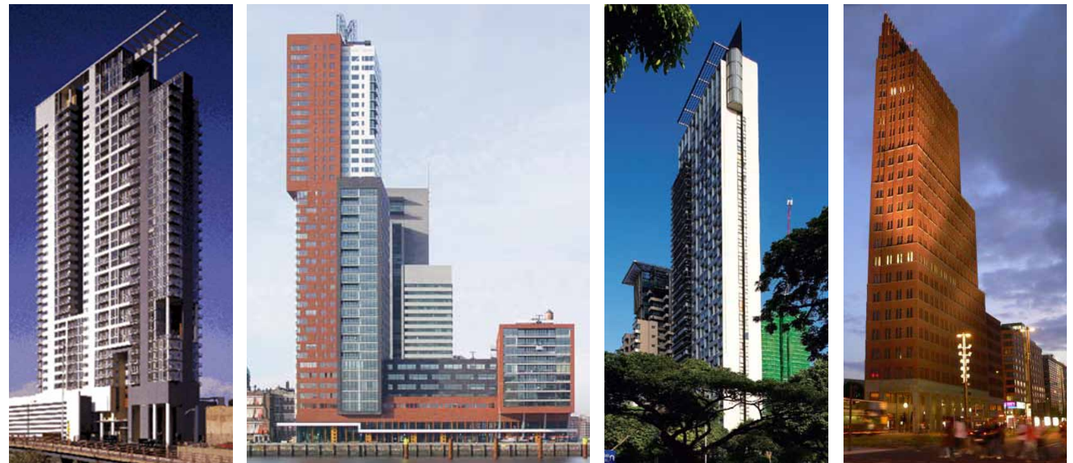
Design towers that create a new identity for the neighborhood with careful articulation of volumes, top, materials palette and building base
