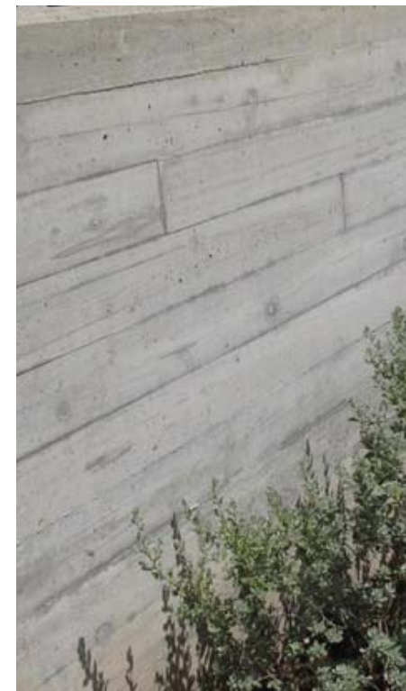
Board Finish Concrete Wall
