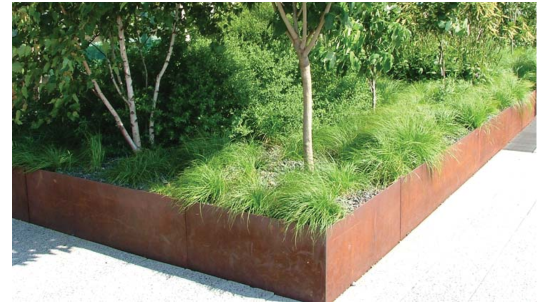
Raised Planting Bed - 18" high segmented metal edging
