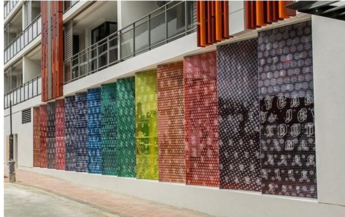
PATTERN PRINTED ON PVB INTERLAYER
