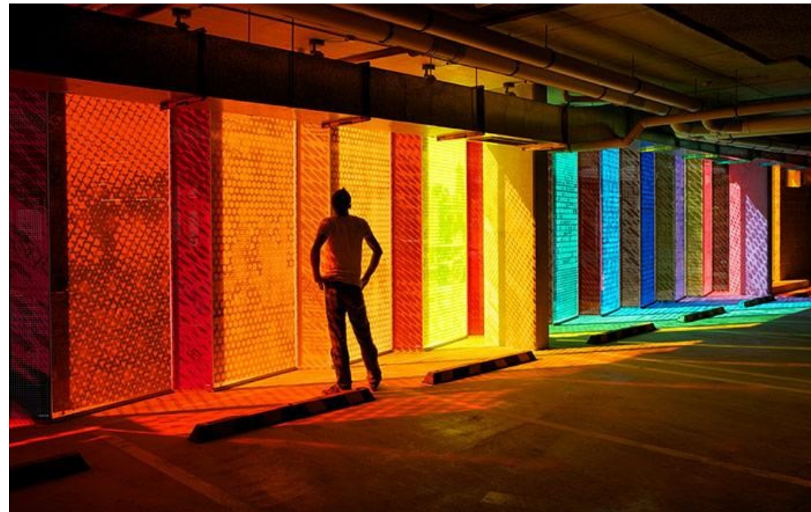
PATTERN PRINTED ON PVB INTERLAYER
