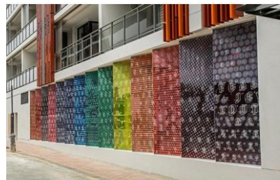
PATTERN PRINTED ON PVB INTERLAYER
