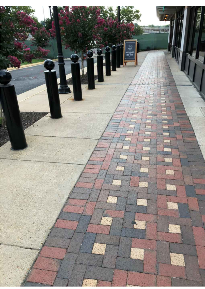
EXISTING CONCRETE AND BRICK PAVER SIDEWALK WEST OF SERVICE DRIVE
