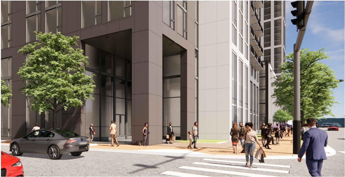
Figure Above: Lobby Entrance at Mill and Eisenhower
