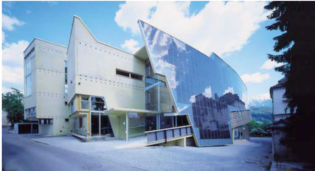
FIG 3: Inclined PV integrated glazed façade of Vocational College in Tirol, Austria
