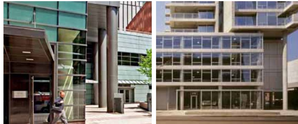
Building base with “Pilotis”
