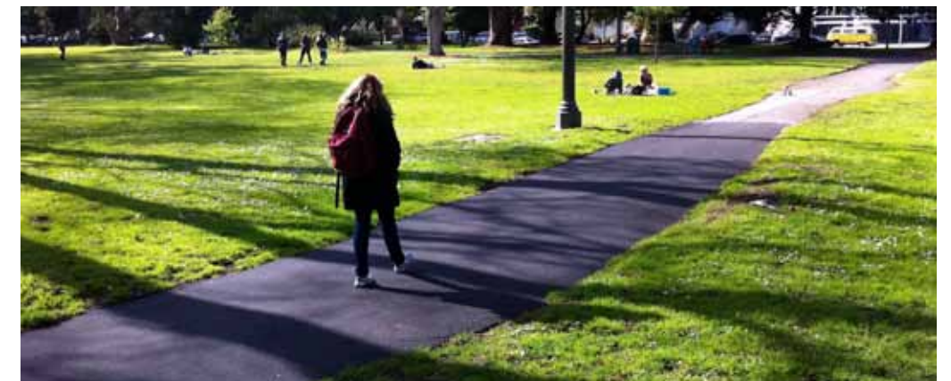
Temporary asphalt walkway
