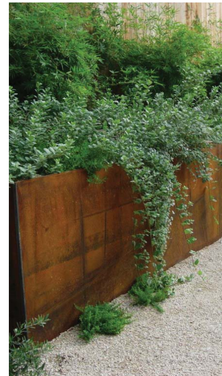
Cor-Ten Steel Walls
