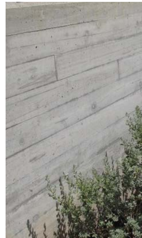
Board Finish Concrete Wall
