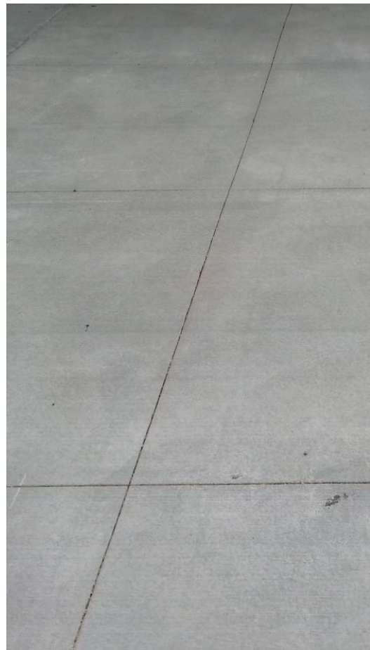
Cast-in-place Concrete Paving - Tinted , w/ Saw cut Joints
