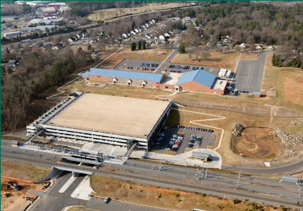
Sterling school/transit parking structure
