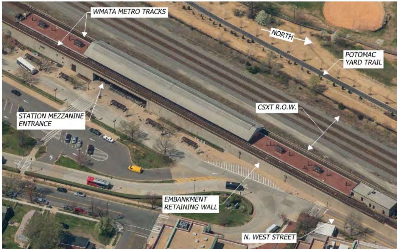
Figure 2: Braddock Road Metrorail Station Site
