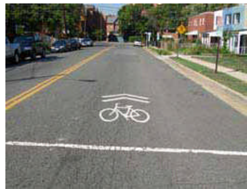
Existing "sharrow" pavement markings on Pendleton Street
