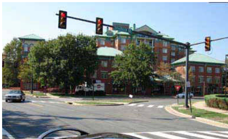
Existing conditions at the Braddock/West/Wythe intersection
