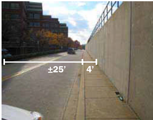
Existing service road behind Braddock Place looking toward Metro
