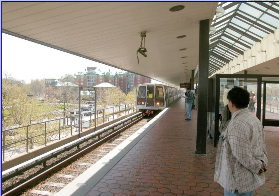
Braddock Road Metro station
