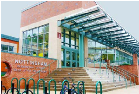
Nottingham Elementary School
