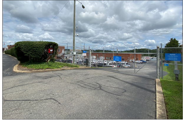
907W Glebe Rd, Dominion Energy (VEPCo) Service Yard, View NW.jpg
