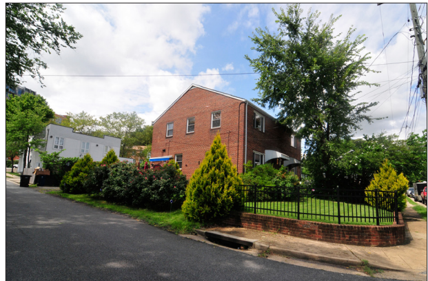
St Elmo Sec 2, 100 Leadbetter and Helen Ave, View SW.jpg
