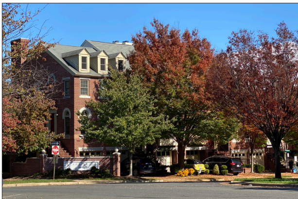
Lenox at Sunnyside, W Glebe Rd and Charles Ave, View NW.JPG
