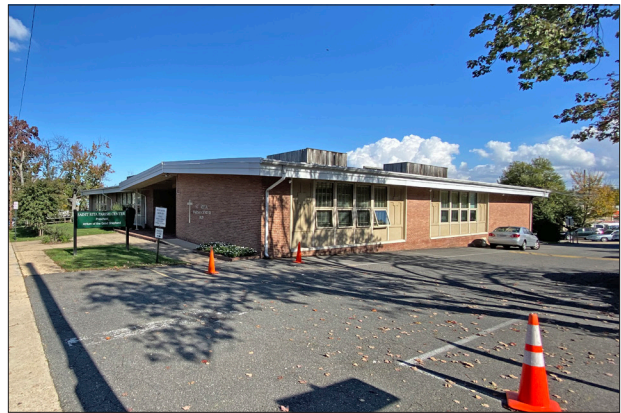
St Rita School Russell Rd added ca 1956, View NE.JPG
