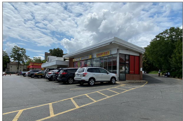
3408 Mount Vernon Ave in front of W&O alignment, View S-SW.jpg
