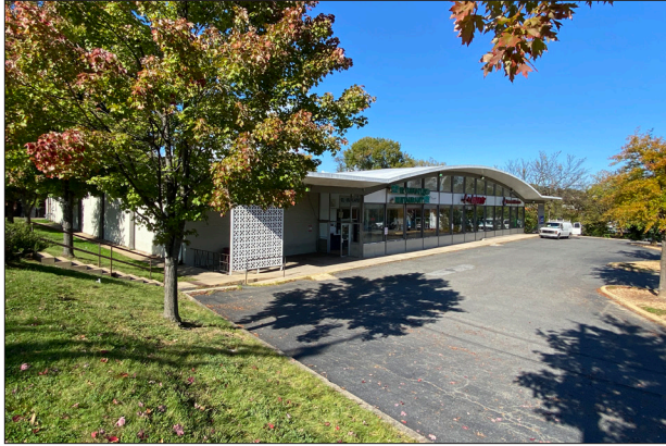
221 W Glebe Rd, View North.JPG
