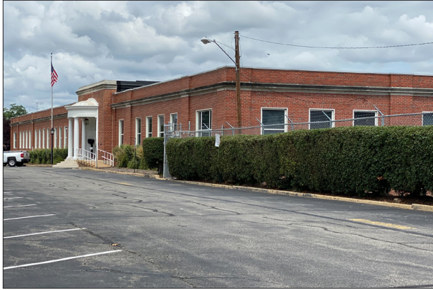
907 W Glebe Rd, Dominion Energy (VEPCo), View NW.jpg
