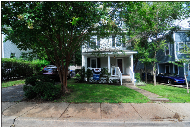
Sunnyside 3814 Elbert Ave, View NW.jpg
