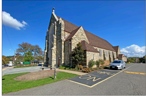
St Rita Church and Rectory, View NE.JPG
