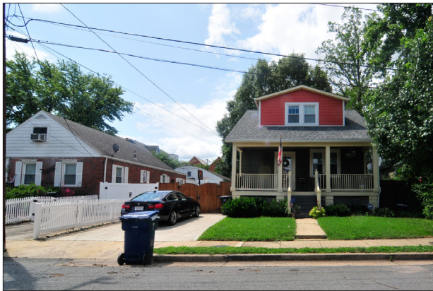
St Elmo Sec 2, 14 Leadbetter Ave, View North.jpg
