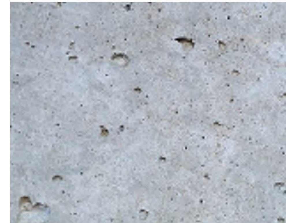
AC01 - EXPOSED CONCRETE
