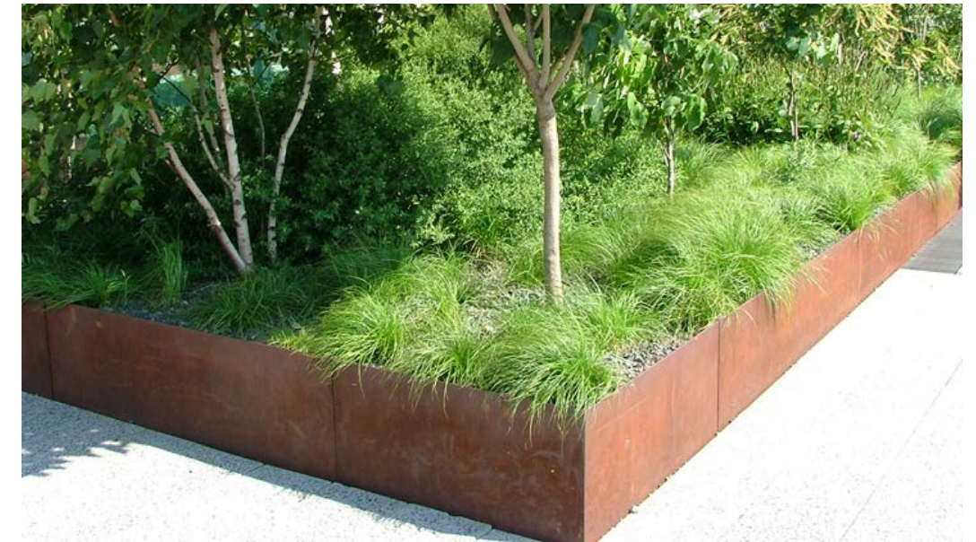
Raised Planting Bed - 18" high segmented metal edging
