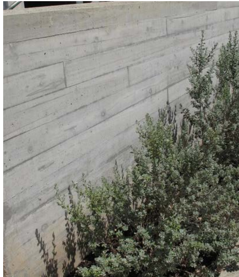
Planter Walls - Poured concrete w/board finish, light gray
