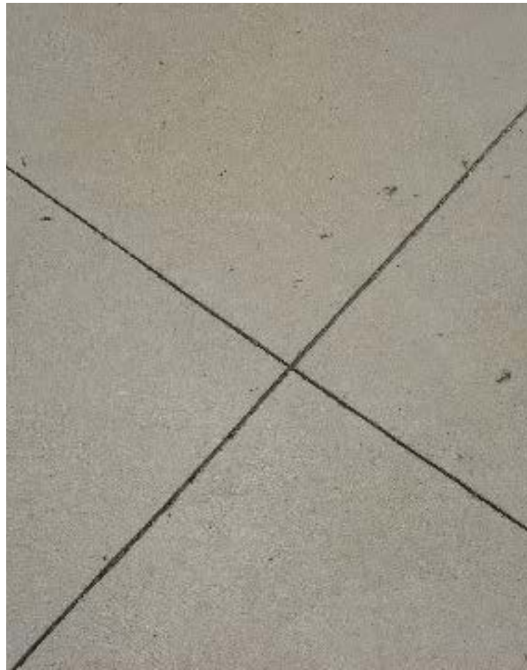
Private Terrace and Stairs - Poured concrete w/ saw-cut joints, med gray
