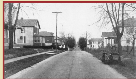
On the eve of annexation in 1929, many of the streets had been paved and lighted, and additional house construction had created a trace town feel to Potomac. Street lighting had been installed in 1910 in the form of forty-five 40-candlepower incandescent lamps. The hard paving of streets began with Mount Vernon Avenue in 1911 and gradually expanded to other streets, although this process was still not complete in 1930. This view shows Hume Avenue from the top of a small ridge, looking east towards Potomac Yard.
