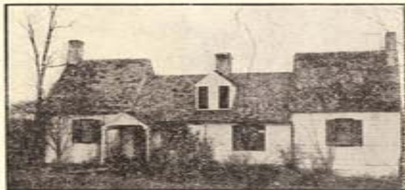
Hollin's Hall Spinning House, Fairfax County.
