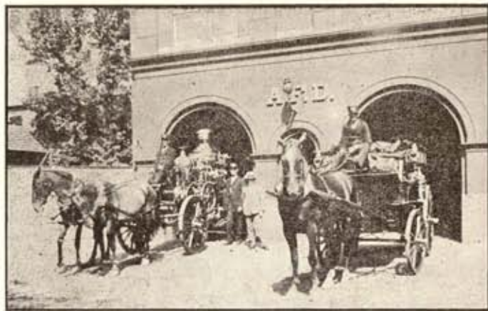
Reliance No. 5 Ready for Service.
