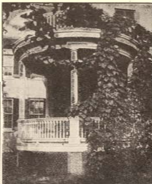
Residence Wm. B. Smoot, rear view.
