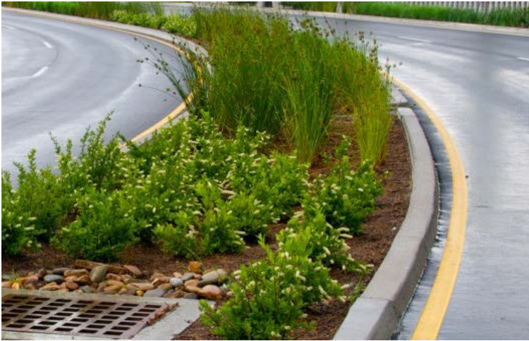
Stormwater management integrated in street design.
