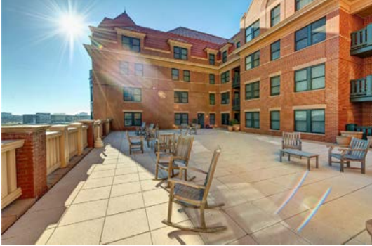
The Station at Potomac Yard residential units amenity area above the Fire Station below.
