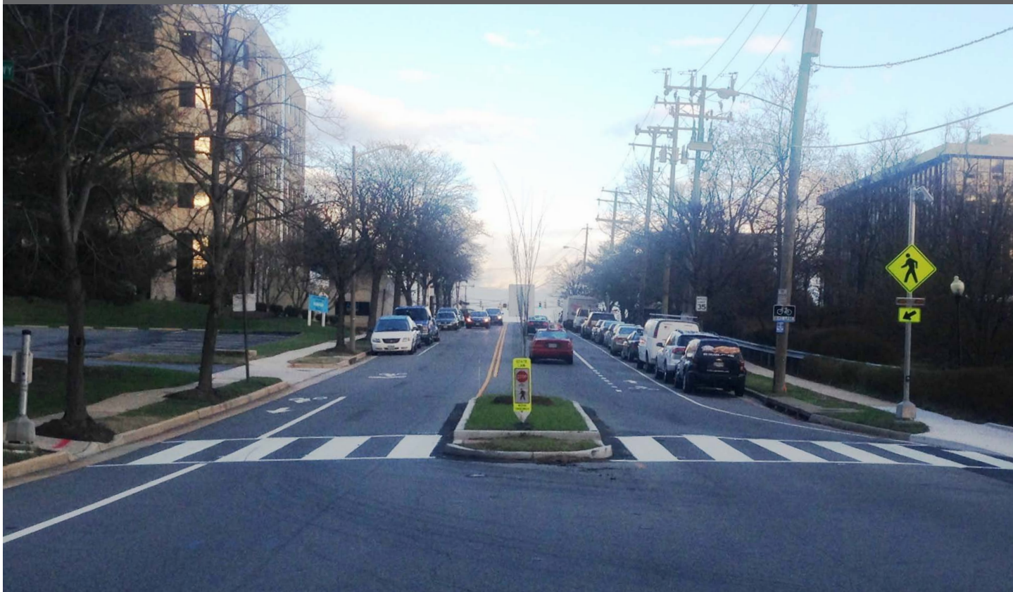
High visibility crosswalk on King Street
