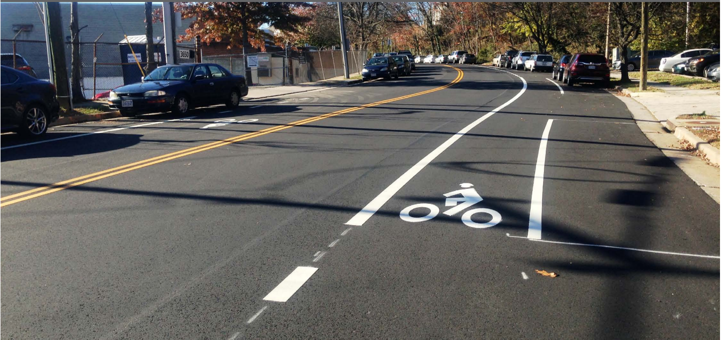
Climbing lane on Wheeler Avenue. Note that there is no lane in the downhill direction.
