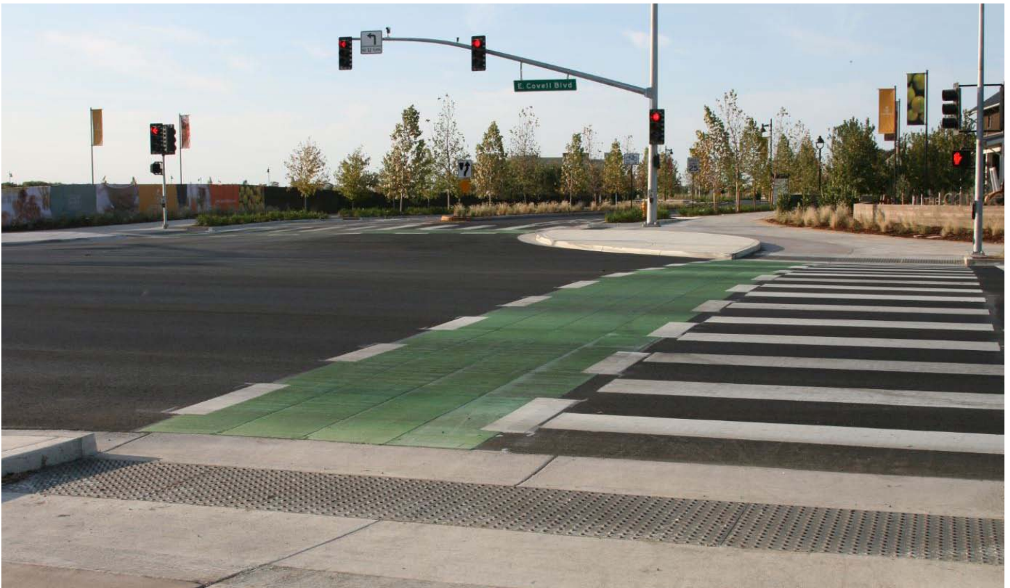
One leg of Davis, CA's protected intersection
