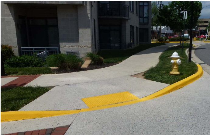
Curb ramp with truncated dome tactile warning
