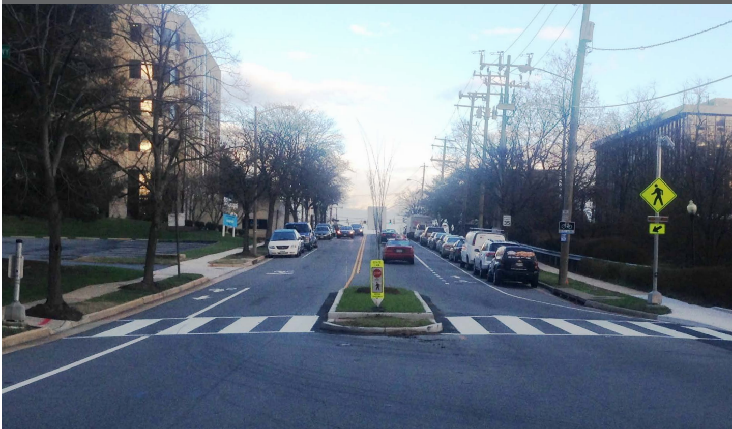
High visibility crosswalk on King Street
