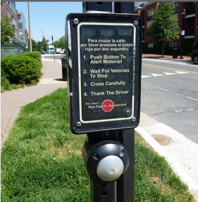
Accessible Pedestrian Signal on Mount Vernon Avenue
