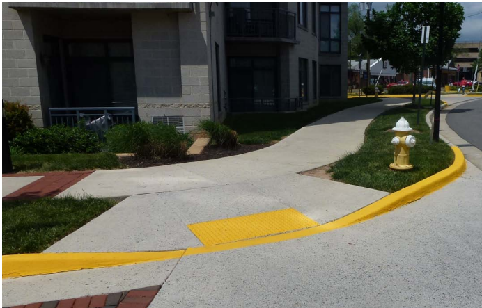
Curb ramp with truncated dome tactile warning
