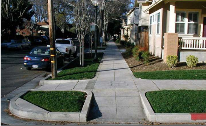
Curb ramp designed without flares. Note: detectable warning strips must be provided
