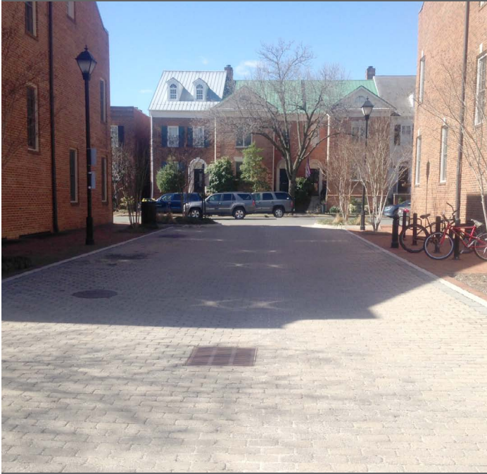
Example of brick paving treatment
