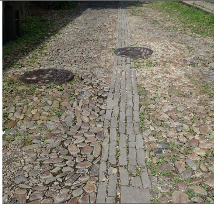
Example of a cobblestone paving treatment
