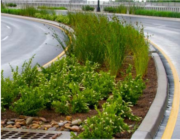
Stormwater management integrated in street design.
