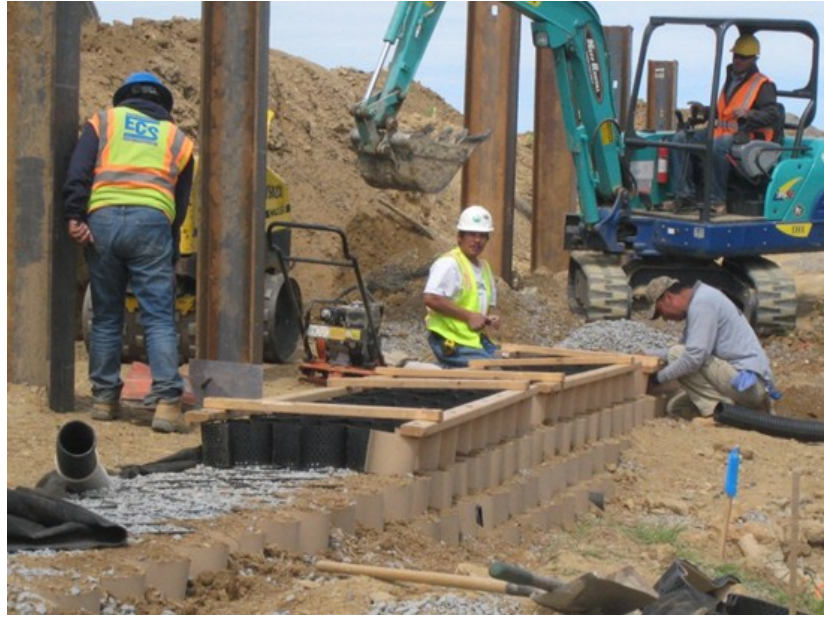
Potomac Yard Park under construction
