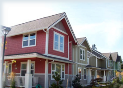
Matthei Place, Bellingham, WA. 14 unit home ownership project of the Kulshan CLT
