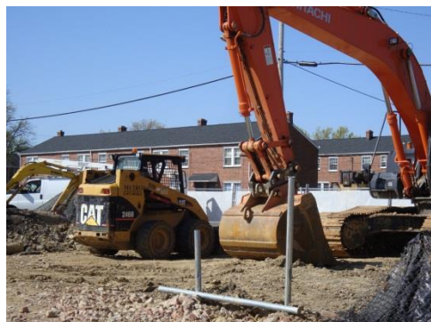
Construction at Old Town Commons
