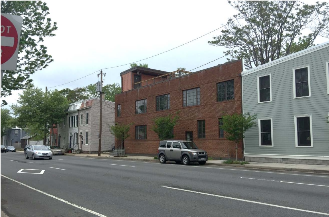
Photograph 27: Pre-1932 contributing buildings on N. Patrick St. south of Ramsey Homes, looking SW from SW corner of N. Patrick and Pendleton St.
