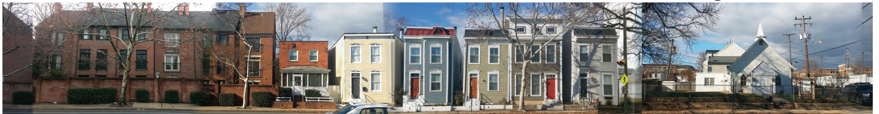
2 LOOKING WEST ON N. PATRICK ST.
