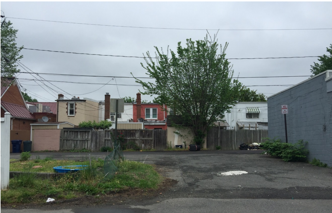
Photograph 24: Rear yards of pre-1932 buildings on N. Alfred St., looking east from Ramsey Homes alley mid-block.
