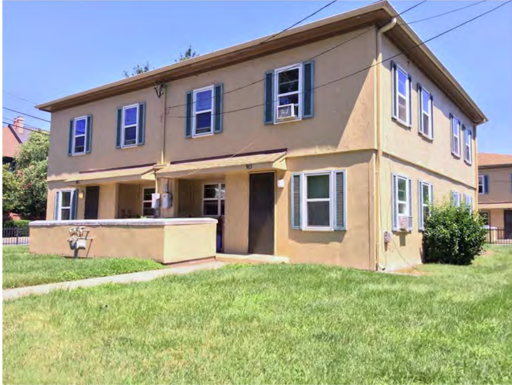
Figure 46: Ramsey Homes, Building IV
