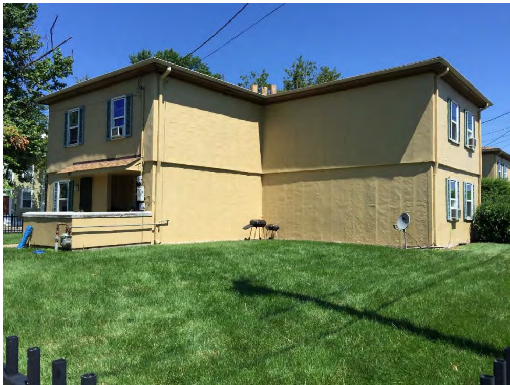
Figure 47: Ramsey Homes, Building II
