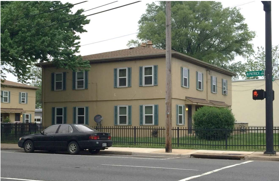
Photograph 14: Ramsey Homes, Buildings IV, looking NE from west side of N. Patrick St.
