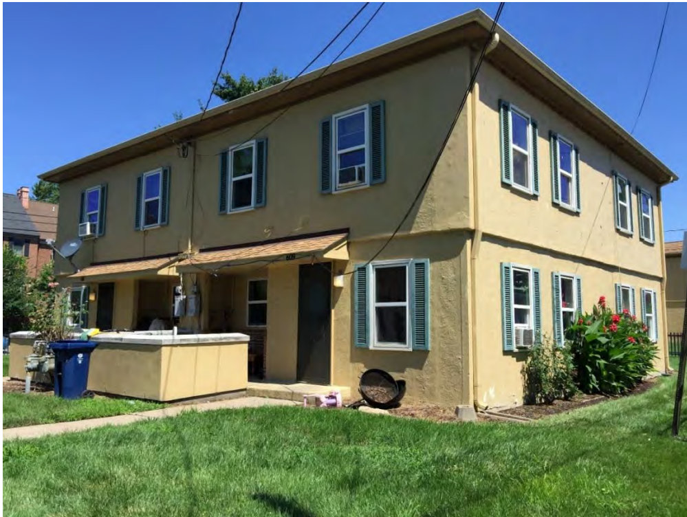
Figure 45: Ramsey Homes, Building III
