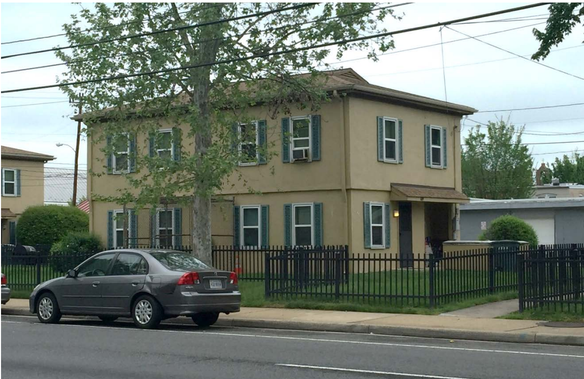
Photograph 12: Ramsey Homes, Buildings II, looking NE from west side of N. Patrick St.
