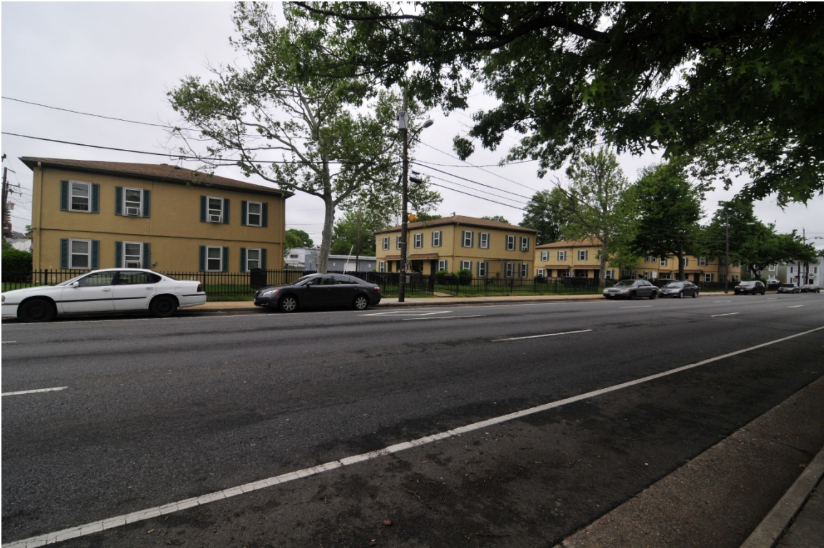
Photograph 7: Ramsey Homes, Buildings I-IV, looking SE from west side of N. Patrick St.
