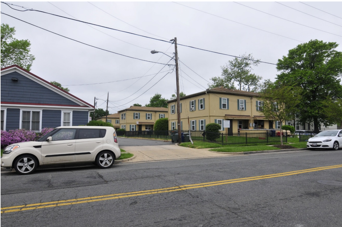
Photograph 4: Ramsey Homes, Buildings I-III, looking south down the alley from north side of Wythe St.
