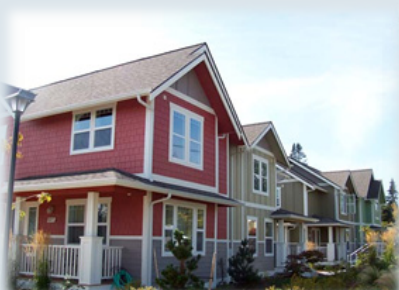
Matthei Place, Bellingham, WA. 14 unit home ownership project of the Kulshan CLT
