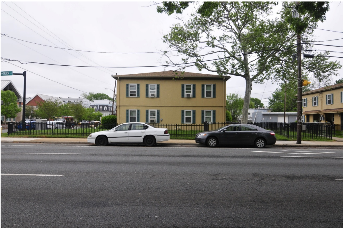
Photograph 10: Ramsey Homes, Buildings I, showing typical side elevation, looking East from West side of N. Patrick St.
