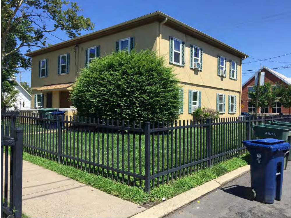
Figure 44: Ramsey Homes, Building I
