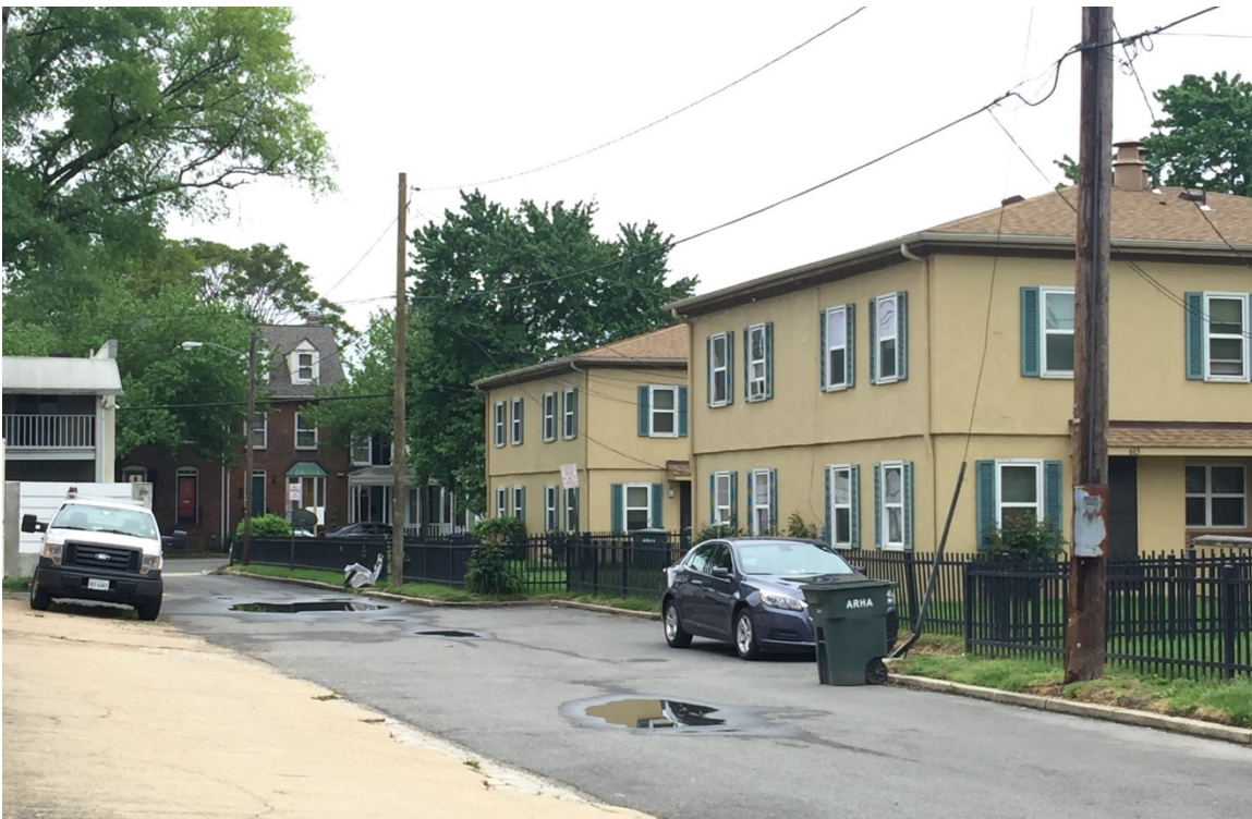
Photograph 16: Ramsey Homes, Buildings IV and III, looking SW from the alley.
