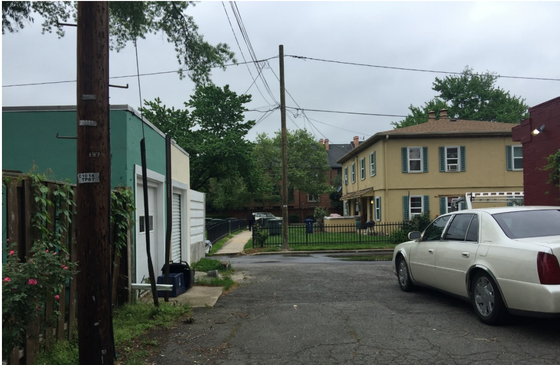
Photograph 21: L to R, Pendleton St. alley garages, King's Rowe (built 1980), and Ramsey Homes Building IV, looking west from N. Alfred St. alley.
