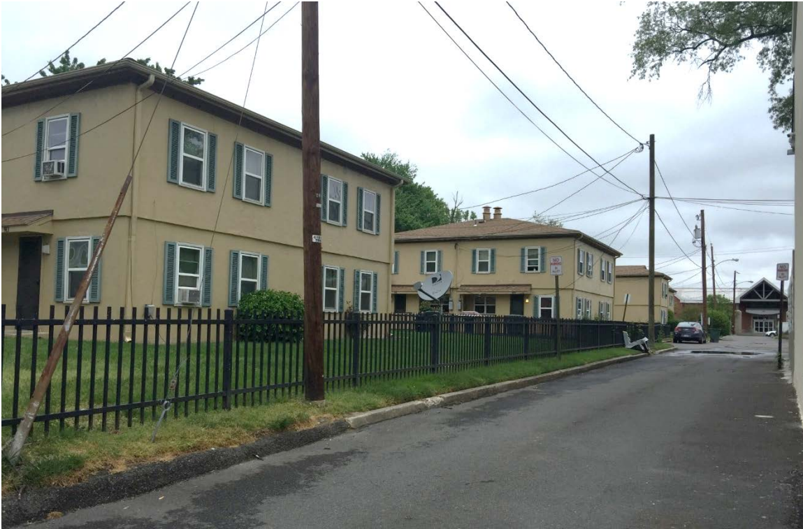
Photograph 15: Ramsey Homes, Buildings IV, III, II, and I and the Rec Center, looking N/NE down the alley from the north side of Pendleton St.
