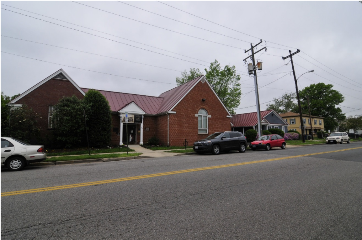
Photograph 1: Alexandria Black History Museum and Ramsey Homes, Building I, looking SW across Wythe St.
