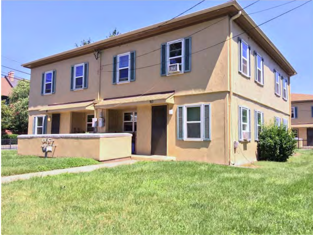
Figure 46: Ramsey Homes, Building IV
