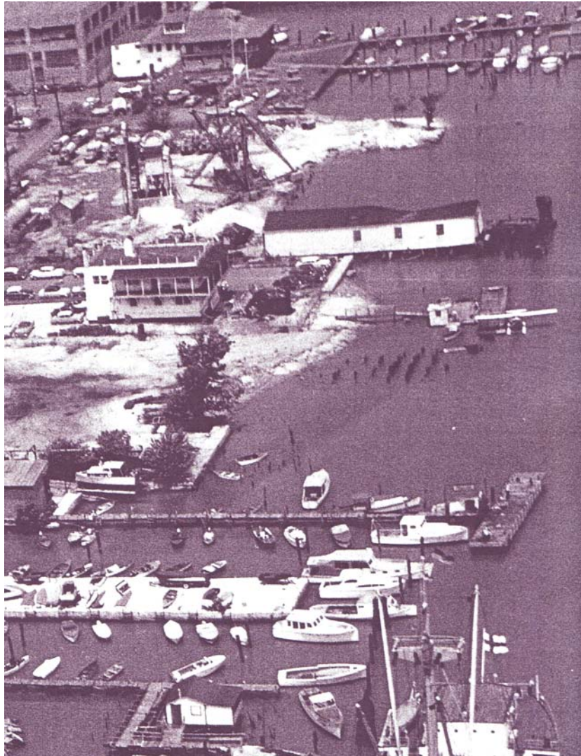
An undated aerial photograph shows the pier Richards builds for restaurant boats, with a floatplane alongside.
