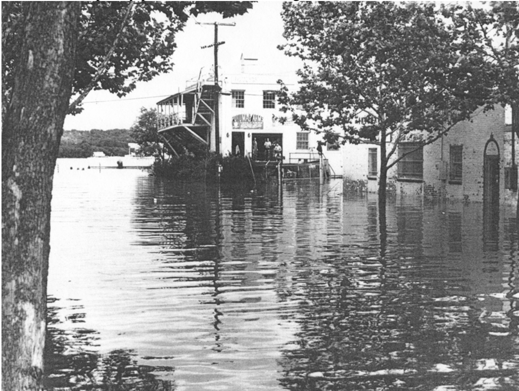
Water once again laps at the concrete pilings in a late 50s or early 60s photo of flooding at Prince and the Strand.
