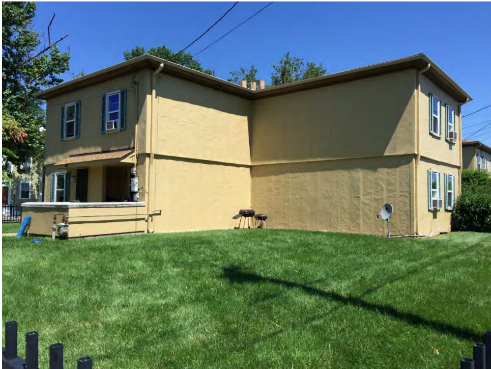
Figure 47: Ramsey Homes, Building II
