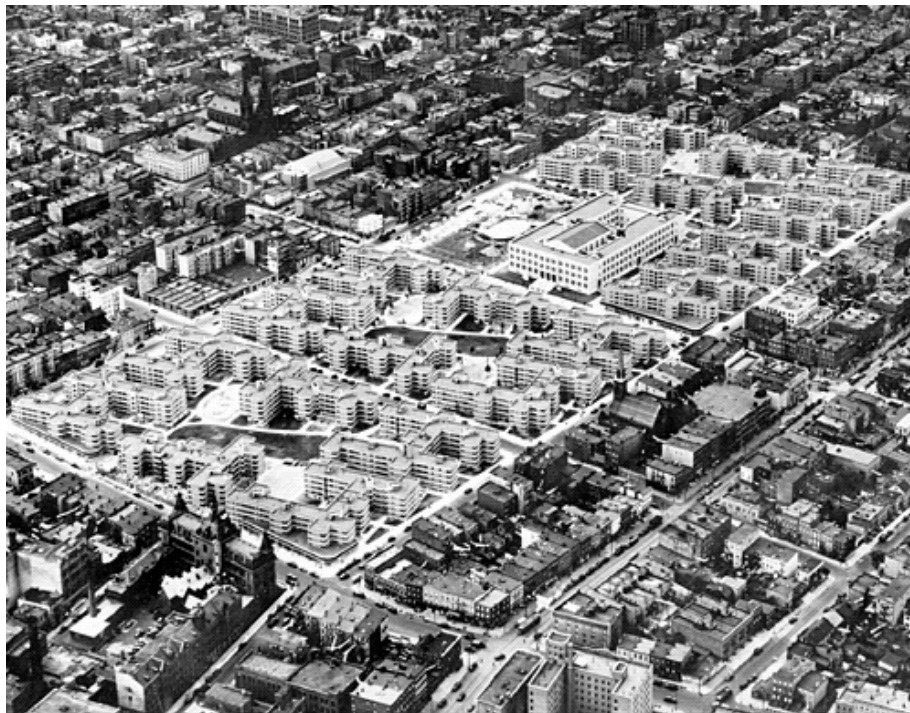
Figure 8: Aerial View of Williamsburg Houses in Brooklyn, New York (Franklin D. Roosevelt Library, National Archives)
