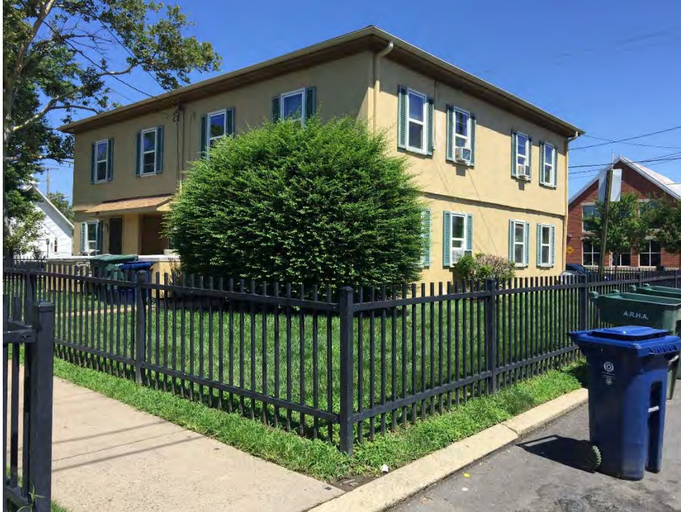
Figure 4: Ramsey Homes, Building I
