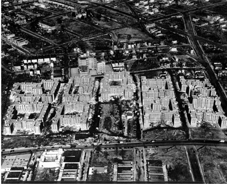
Figure 22: Aerial View, PWA Built Hillside Homes, Bronx, New York (Franklin D. Roosevelt Library, National Archives)
