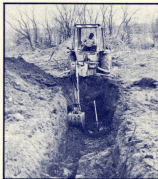
4. Uncovering the Pool No. 1 south wall which is composed of large, dry laid stones.
