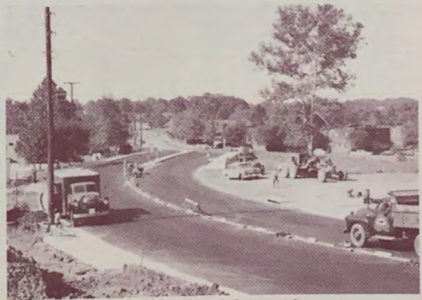
Bridge at Glebe Road
