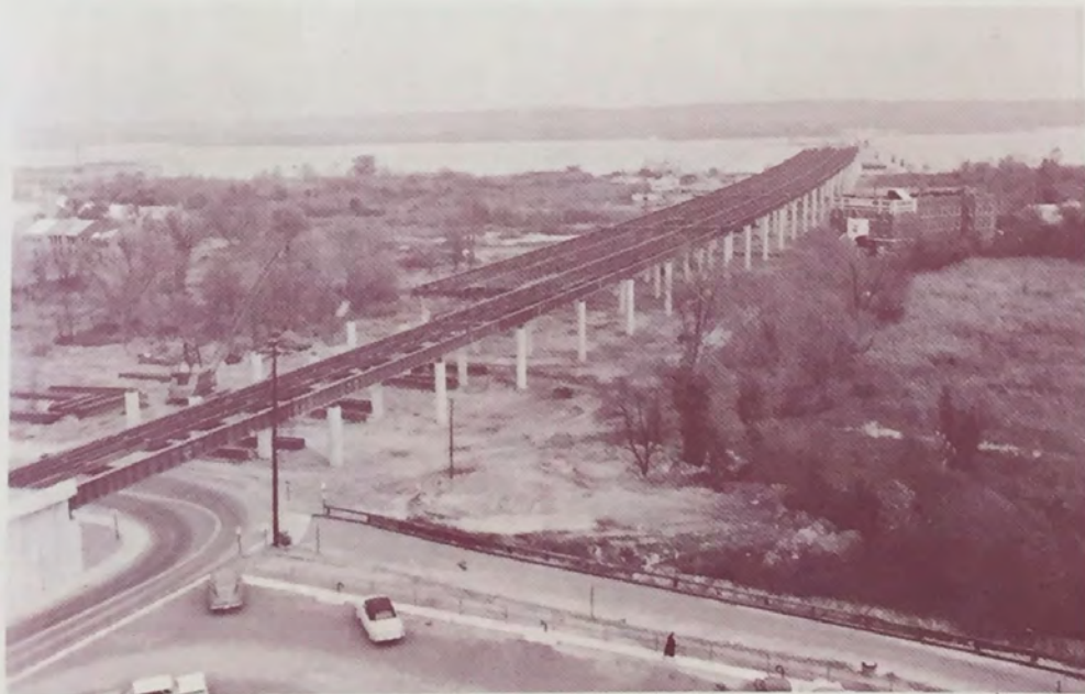
Woodrow Wilson Bridge
