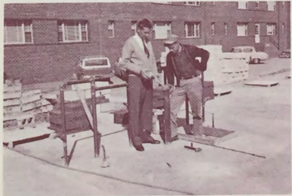
Plumbing Installation Inspection
