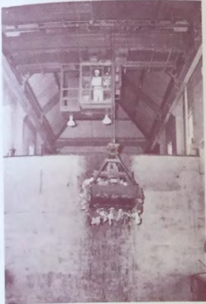
Overhead Crane at the Incinerator
