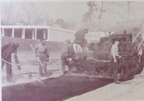
Street Construction Valley Drive
