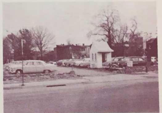
Alfred St. under construction
