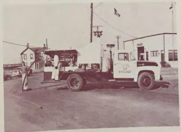
Sewer Maintenance Equipment
