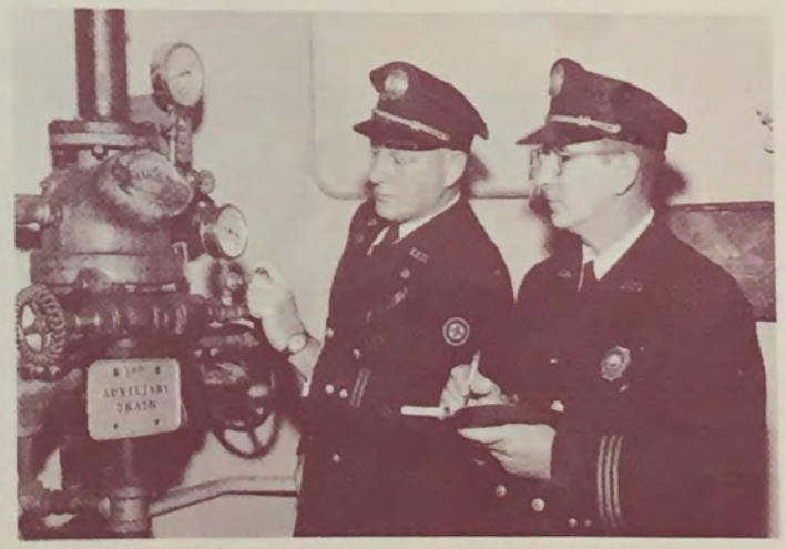
Inspection of Automatic Sprinkler System
