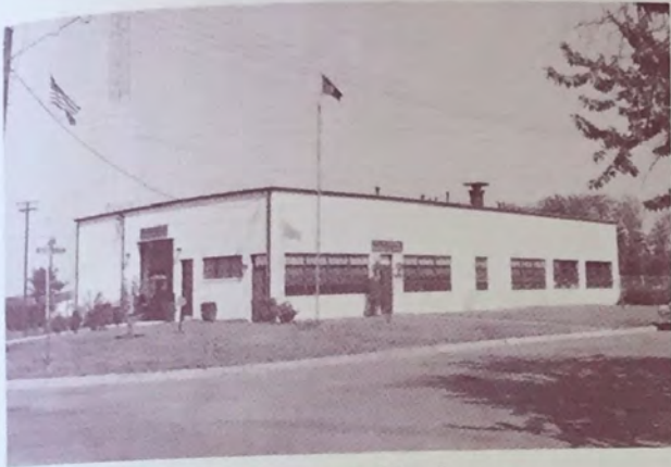
Traffic Department Headquarters
