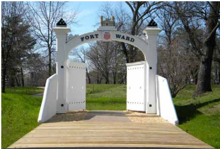
Fort Ward Reconstructed Gate
