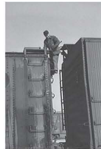
Before car retarders, brakemen slowed cars manually. Courtesy of The Library of Congress.
