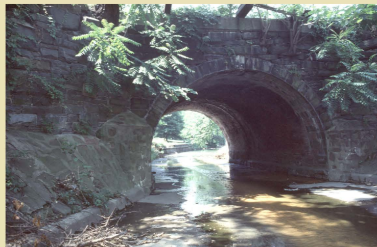
The north face of the original stone bridge is in smooth and rock-faced gray sandstone laid in random-range ashlar; the stone may have come from the Little Falls of the Potomac. Alexandria Archaeology Museum
