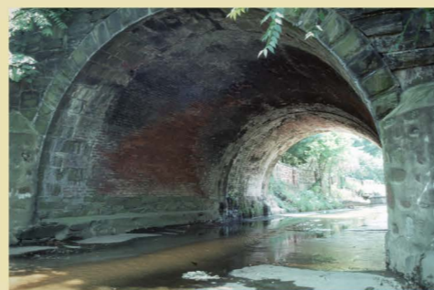
The brick barrel vaults of both the original stone bridge and the southern addition are laid in all-stretcher bond; the semicircular arch spans 21 feet 1 1/2 inches and rises 10 feet 6 inches. Alexandria Archaeology Museum
