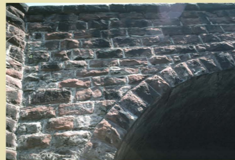
The southern addition to Hooffs Run Bridge constructed of red Seneca Sandstone has an arch composed of 33 rock-face ashlar voussoirs and a larger keystone. The east wing wall descends on top of the Alexandria National Cemetery wall, which is made of similar stone. Alexandria Archaeology Museum
