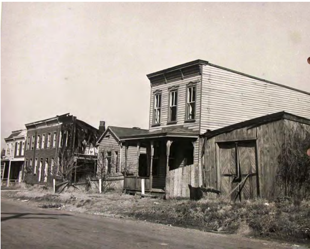
North Side of the 800 Block of Madison Street, View to Northwest: 1940s
