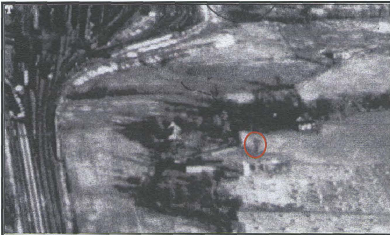
Figure 4. Part of a 1927 aerial view of western Alexandria, showing Cameron Farm in relation to the Southern Railroad yards. Red circle indicates approximate location of vault (Courtesy of Virginia Room, Kate Waller Barrett Branch, Alexandria Public Library)
