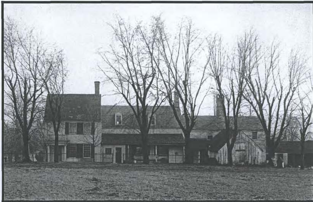
Figure 57. North façade of principal dwelling at Cameron Farm during the late nineteenth century, showing telescoped arrangements of building components and the icehouse structure (far right)(orientation south) (Special Collections, Alexandria Public Library)
