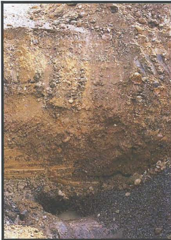
Figure 13. Block 4, Trench 3: Profile of east wall at 400 ft north, showing unconsolidated fill deposit and terra cotta drain pipe and water seepage
