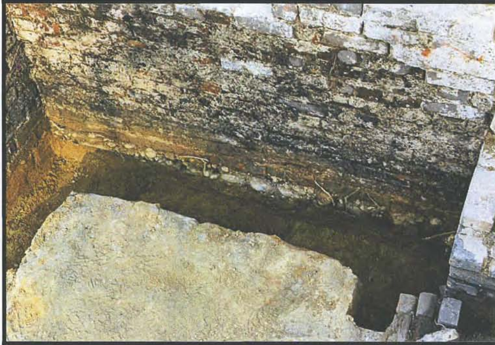
Figure 73. Test Unit 16, west wall, main house, showing brick pier as independent architectural element
