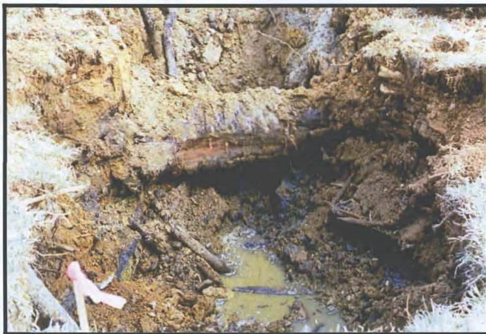
Figure 51. Hoffman property, Trench 10/1.01: General photograph of excavation, showing depth and nature of fill overburden
