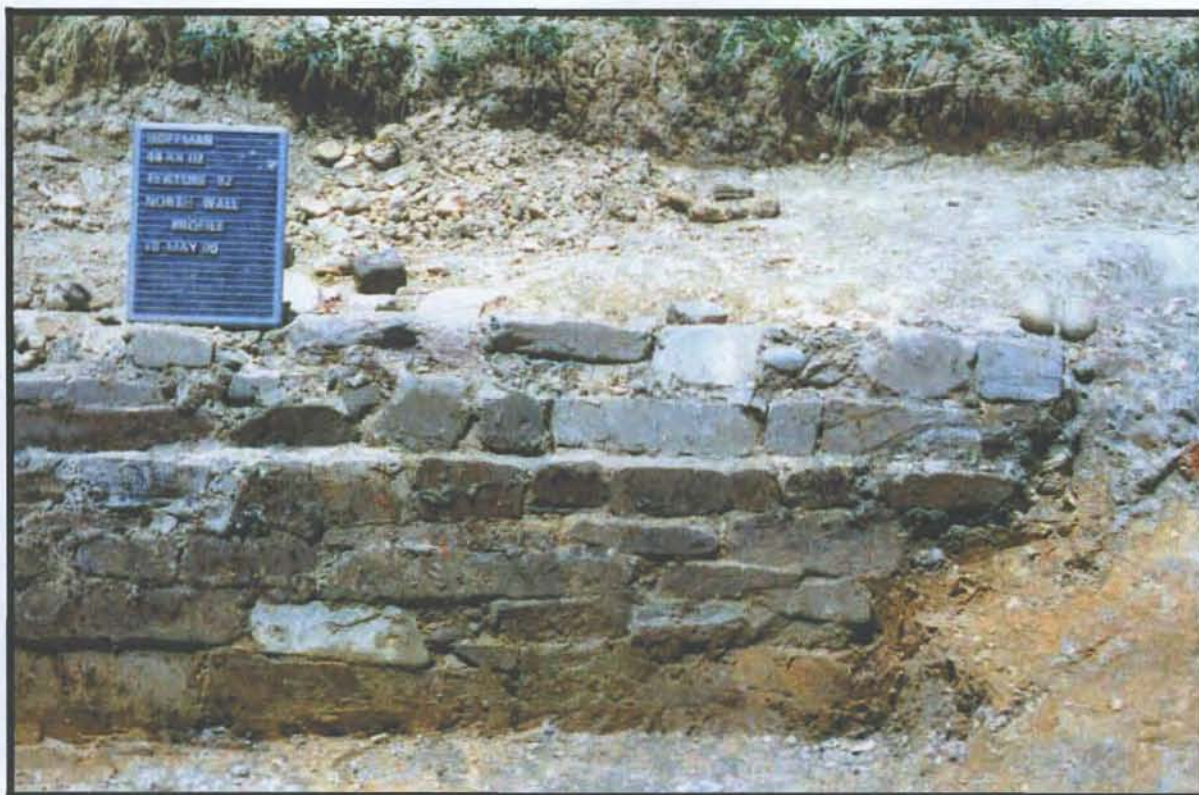
Figure 97. Photograph of the northern stone foundation of the Miller's House (Feature 82), showing coursed ashlar construction, and stepped-back top sections
