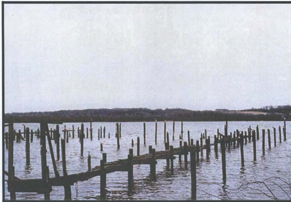
Figure 56. Remnant piers/wharves for small craft: Potomac waterfront at foot of Gibbon Street, Alexandria, Virginia
