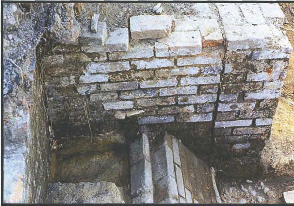
Figure 75. Test Unit 14: Detail of east wall, bulkhead entrance, showing the lower “ramp” feature, and the junction between the main house foundation and bulkhead wall
