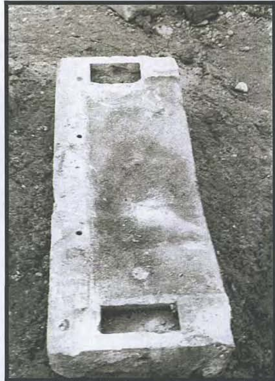
Figure 71. Detail of stone step recovered from rubble fill in the basement of the main dwelling at Cameron Farm, showing mortise holes for insertion of railings
