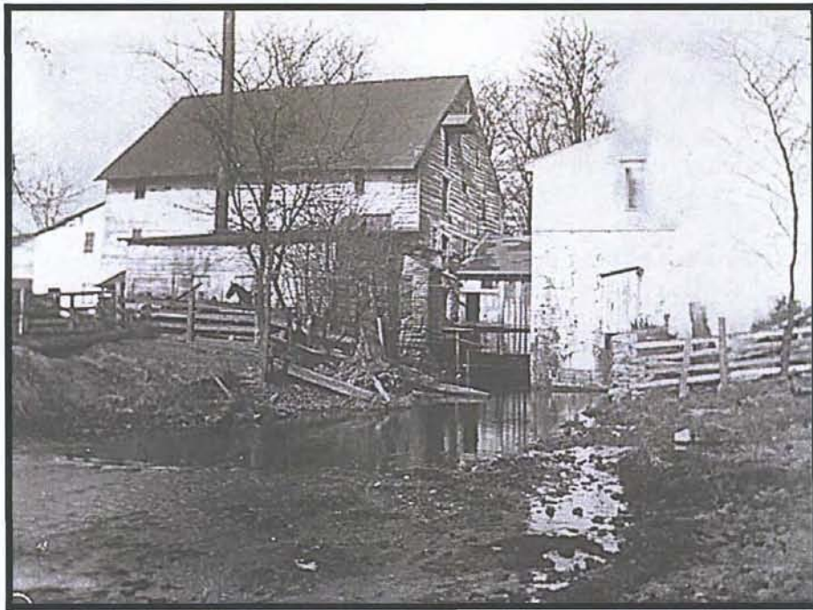
Figure 34. Ca. 1889 view of Cameron Mill and the Alexandria Water Company's pump house (orientation north) (Special Collections, Alexandria Public Library)
