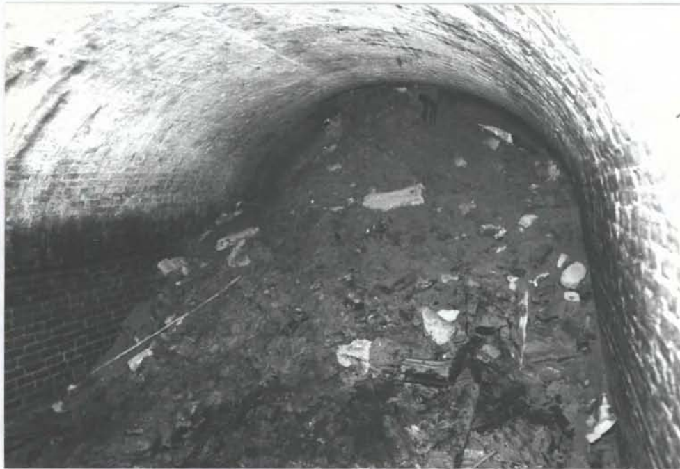
Structure 1 interior showing fill pile, facing south
