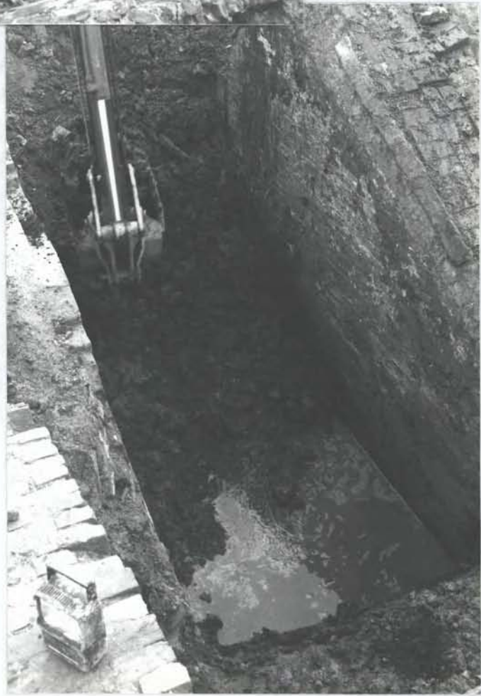
Excavation of Structure 2, interior facing east
