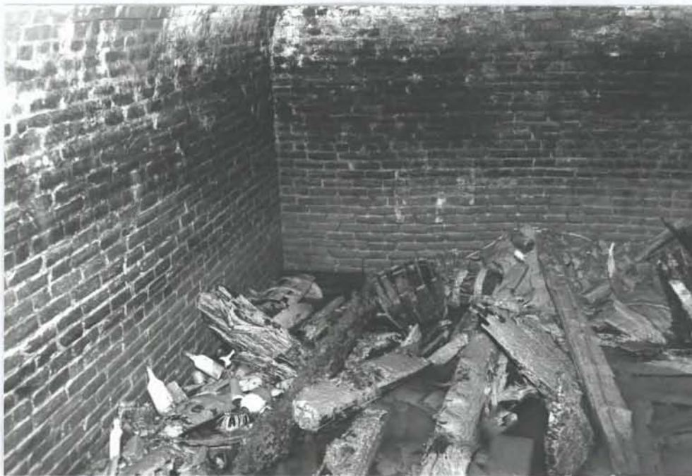
Structure 1 interior, northwest corner
