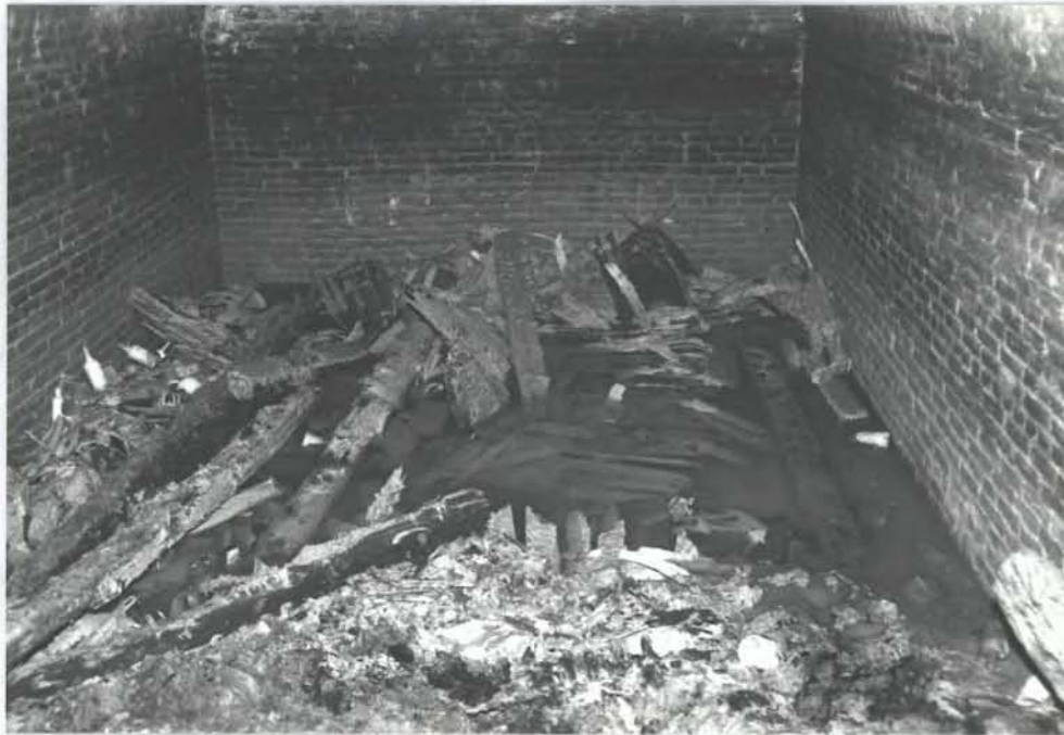
Structure 1 interior, facing north
