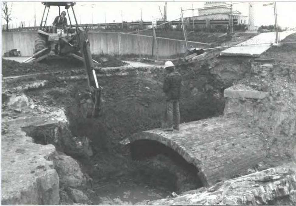
Excavation of Structure 2, facing west
