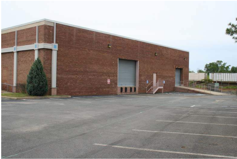
PLATE 35 Building 2 and Surroundings on the Braddock Gateway Property, View to Southwest
