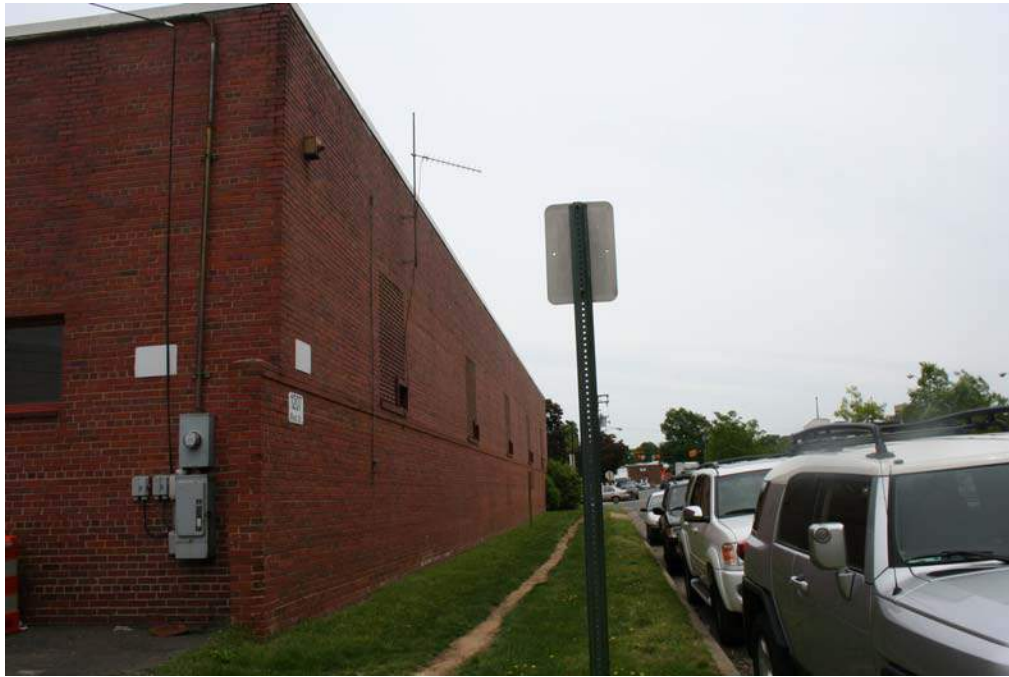
PLATE 41 Building 4 and Surroundings on the Braddock Gateway Property, View to Northwest
