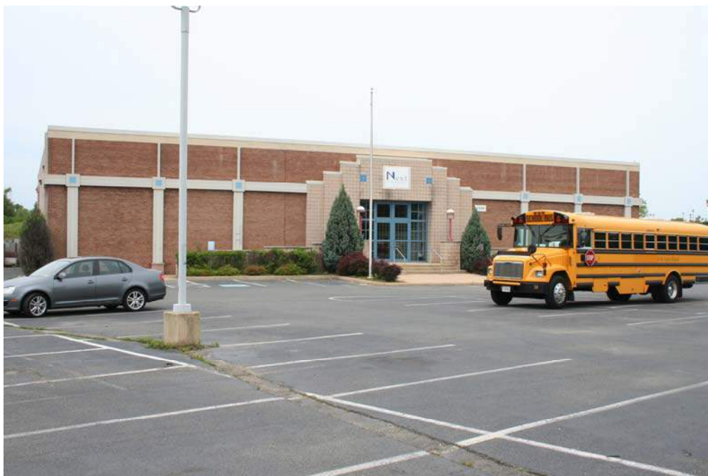
PLATE 34 Building 2 and Surroundings on the Braddock Gateway Property, View to West
