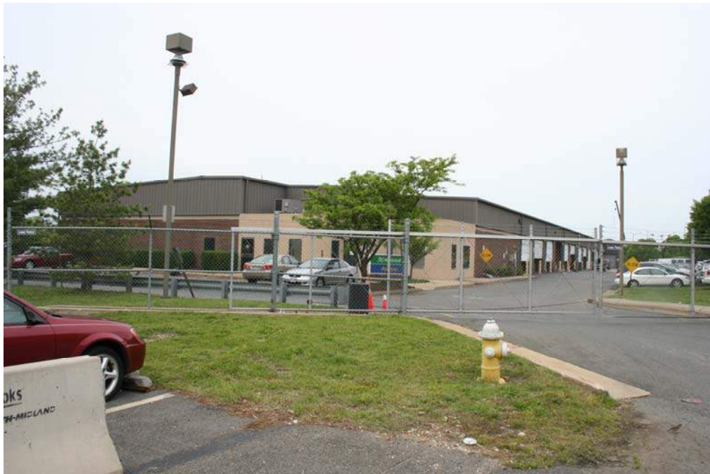
PLATE 32 Building 1 and Surroundings on the Braddock Gateway Property, View to North
