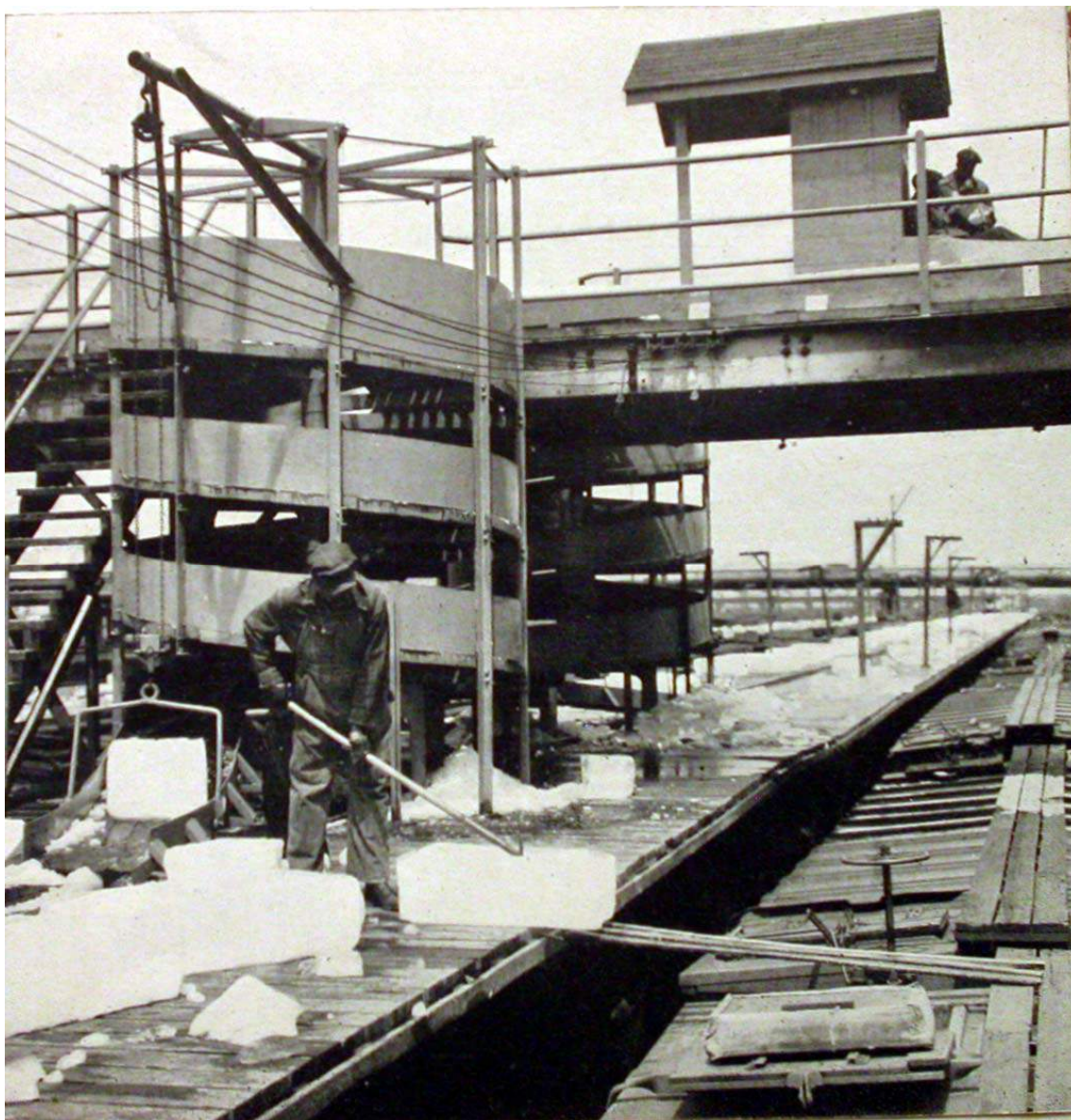
PLATE 26 Mutual Ice Company Icing Operation; Note Spiral Ice Chute; Adapted from Esso Oilways , 1946
