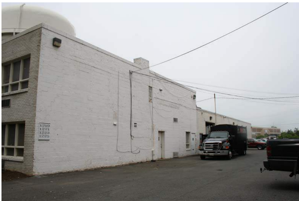
PLATE 38 Building 3 and Surroundings on the Braddock Gateway Property, View to Northwest
