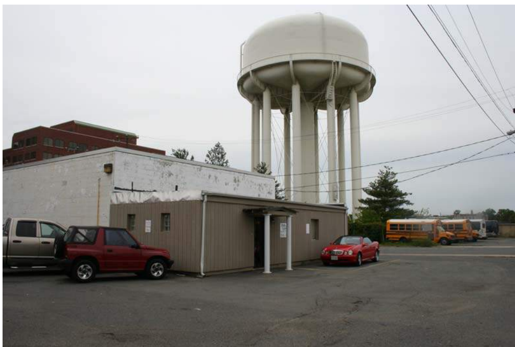
PLATE 39 Building 3 and Surroundings on the Braddock Gateway Property, View to Southwest
