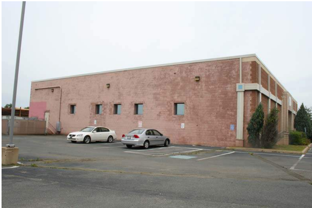
PLATE 36 Building 2 and Surroundings on the Braddock Gateway Property, View to Northwest
