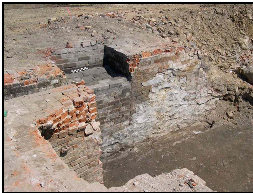
Figure 89. Photograph of the modification to the northern wall of the cellar
