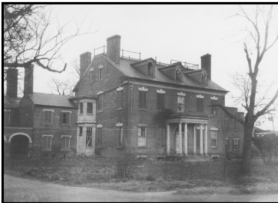
Figure 12. Post-1918 photograph of Colross, following Smoot sale of the property, showing deteriorating condition of house (Courtesy, Special Collections, Alexandria Public Library)
