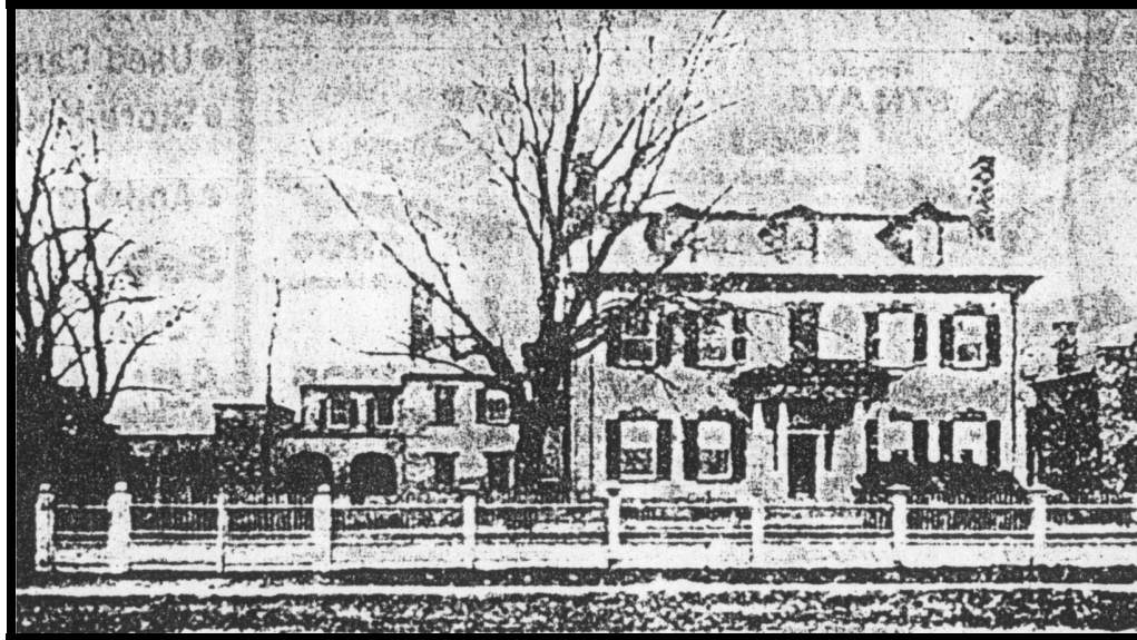
Figure 10. Late nineteenth or early twentieth century photograph of Colross house, showing possible brick and wrought iron fence and dark-colored lintels and window sills (Courtesy, Special Collections, Alexandria Public Library)
