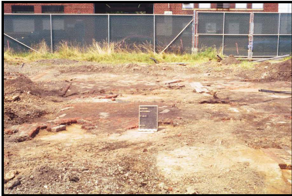
Figure 79. Photograph of the stable foundation
