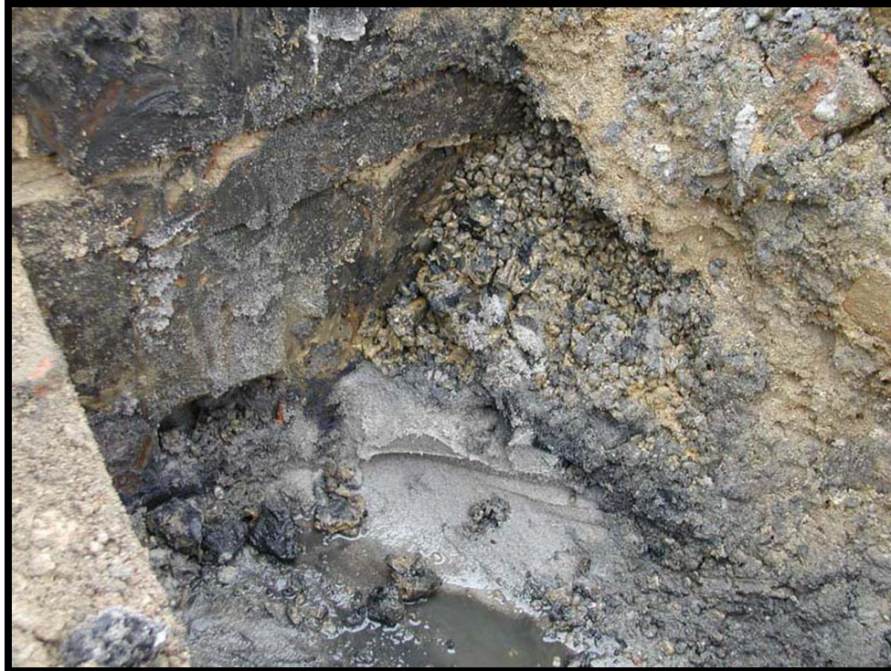
Figure 92. Photograph of the filtration materials for the cistern
