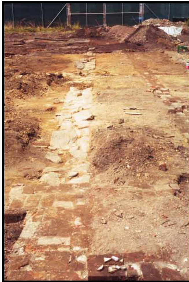
Figure 77. Photograph of the foundations of the dependency buildings
