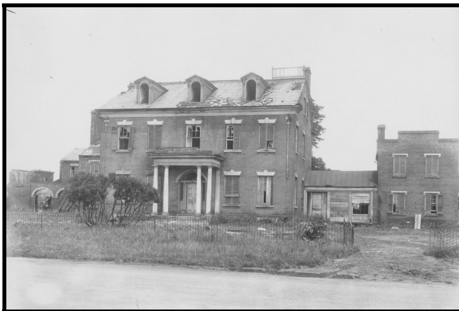
Figure 13. Post-1927 photograph of Colross, showing damage wrought by tornado (Courtesy, Special Collections, Alexandria Public Library)
