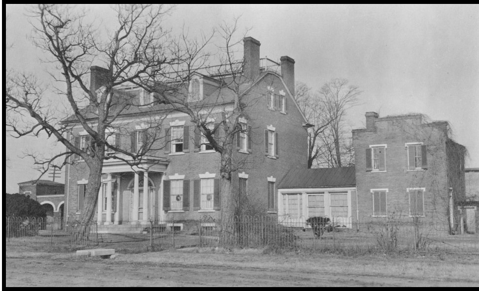
Figure 7. Photograph of Colross, taken approximately 1906, showing the east wing with its connecting hyphen, both added during the Mason period (Courtesy, Special Collections, Alexandria Public Library)
