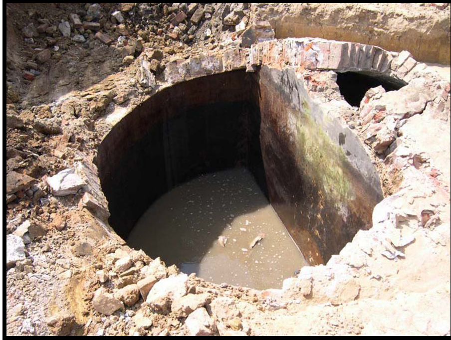
Figure 75. Photograph of the interior dividing wall of the cistern
