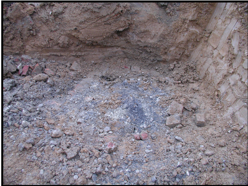
Figure 98. Photograph of the well shaft at the base of excavations
