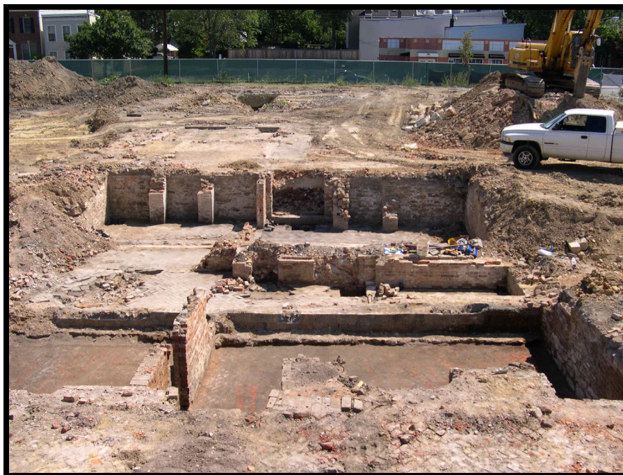
Figure 82. Overall photograph of the exposed cellar showing the eastern, central and western portions; photo direction: east
